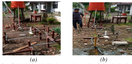
Gambar 3. Model instalasi jaringan pipa (a) pipa Galvanis (b) pipa HDPE
